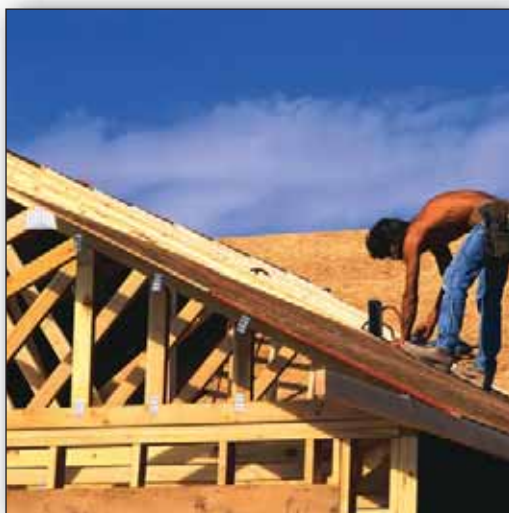
Permanent bracing system
