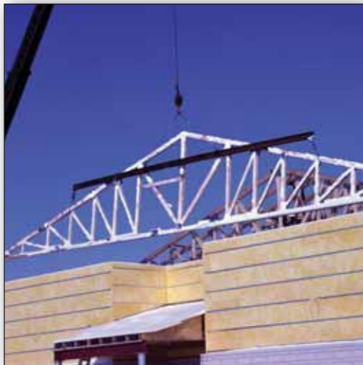
Erecting the trusses on the jobsite
