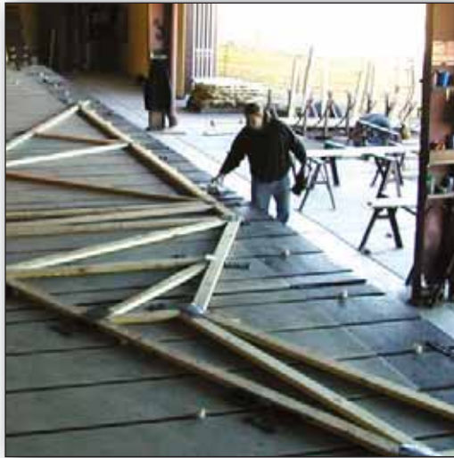
Manufacturing the trusses
